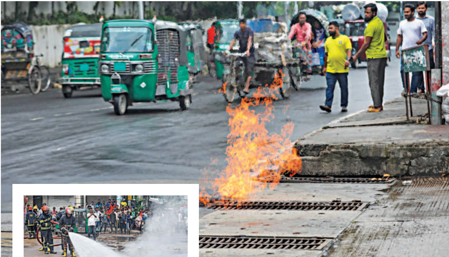
Flames shoot up from an underground gas pipeline after it burst on Zakir Hossain Road in the Foy's Lake area of Chattogram city yesterday afternoon, triggering panic among pedestrians and vehicle passengers. Fire service personnel brought the blaze under control after about an hour and a half of effort.
