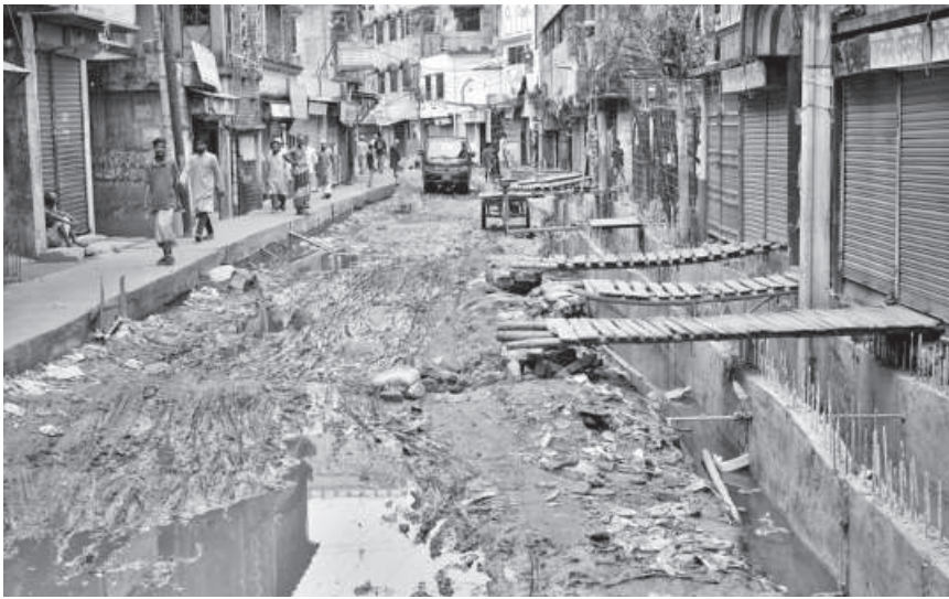
Ongoing drain construction has left a road in Shyampur's Uttar Jurain area muddy and difficult to use, causing suffering to residents and pedestrians. Makeshift bamboo walkways have been placed over the open drain so people can access nearby shops and houses.
