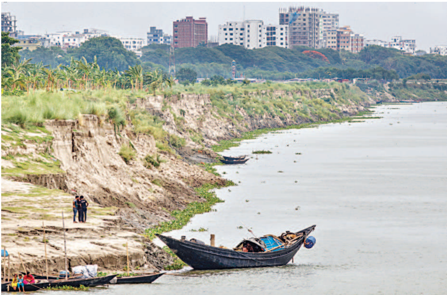
Erosion along the Padma river is threatening Rajshahi city, with large stretches of the riverbank collapsing and the water advancing towards homes and urban infrastructure. Despite government protection efforts, seasonal fluctuations in water levels continue to accelerate land loss. The photo was taken recently.
