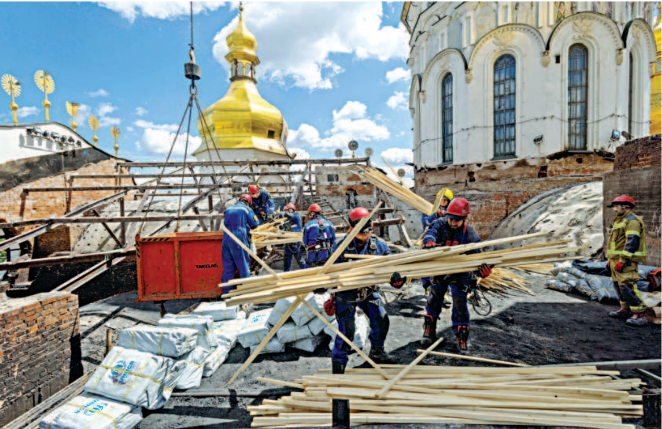
Ukrainian workers repair the roof of the Dormition Cathedral at the Kyiv Pechersk Lavra after it was damaged in Russian missile and drone strikes yesterday.
