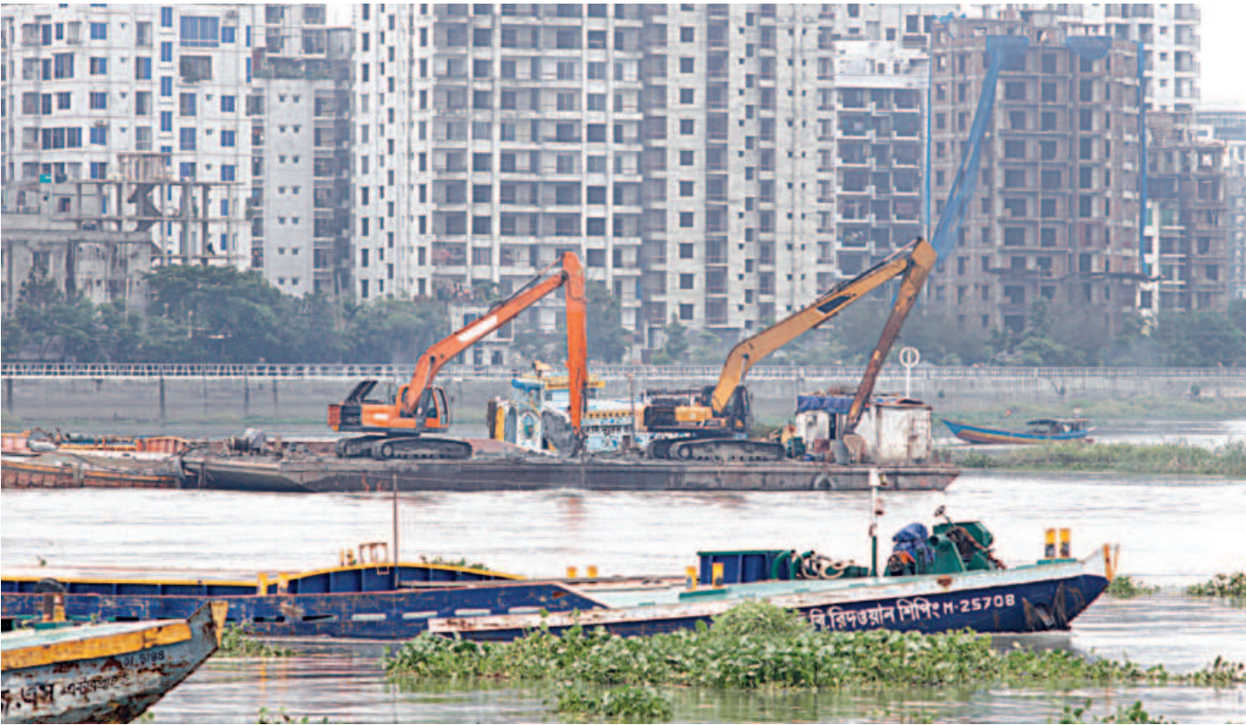
Heavy excavators mounted on barges are lifting soil and sand from the Turag river in the Ramchandrapur area of Dhaka. Local influentials are reportedly extracting sand illegally from the riverbed to sell to brick kilns, contributing to significant environmental degradation and riverbank erosion. The photo was taken yesterday morning.
