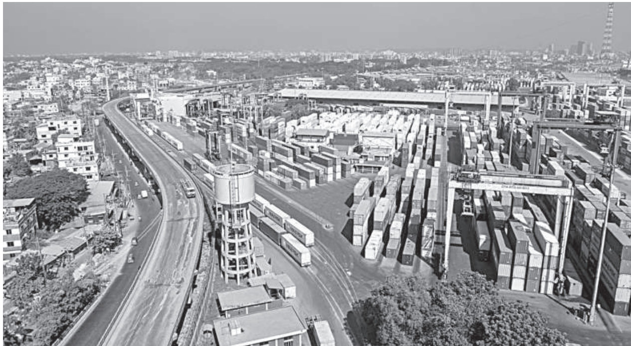
Ports are complex infrastructures tied to not only trade performances, but also social well-being and environmental resilience.'
