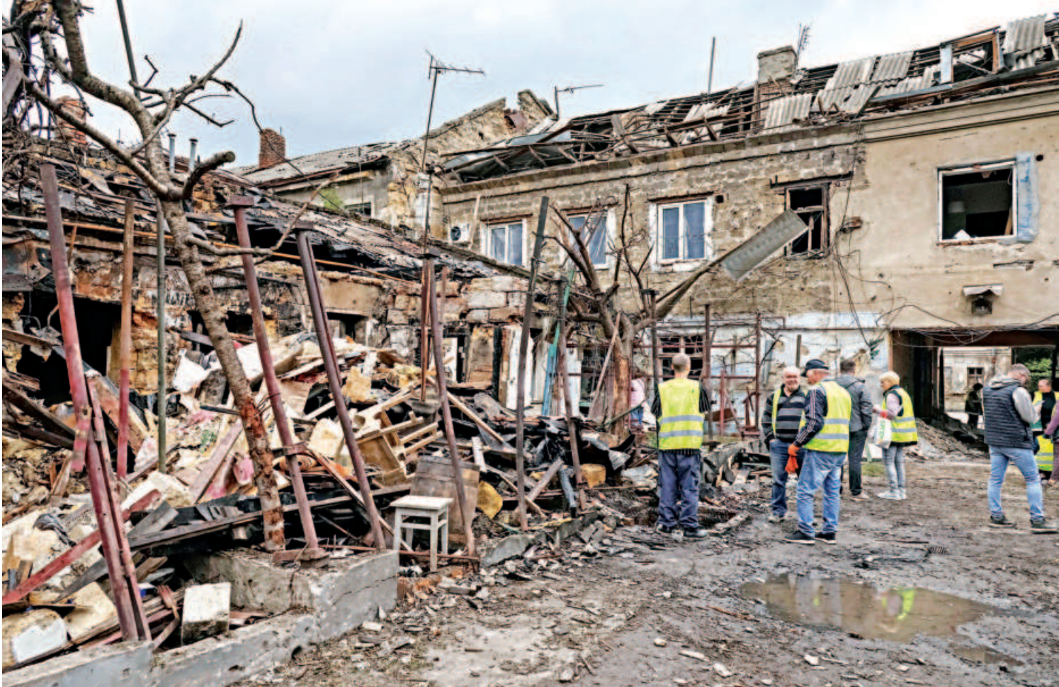
Community workers stand at the site of an apartment building and houses damaged by a Russian drone strike in Odesa, Ukraine, yesterday. Russia fired a record number of long-range drones at Ukraine in May, an AFP analysis of Ukrainian air force data showed, as Kyiv appealed to allies for air defence support.
