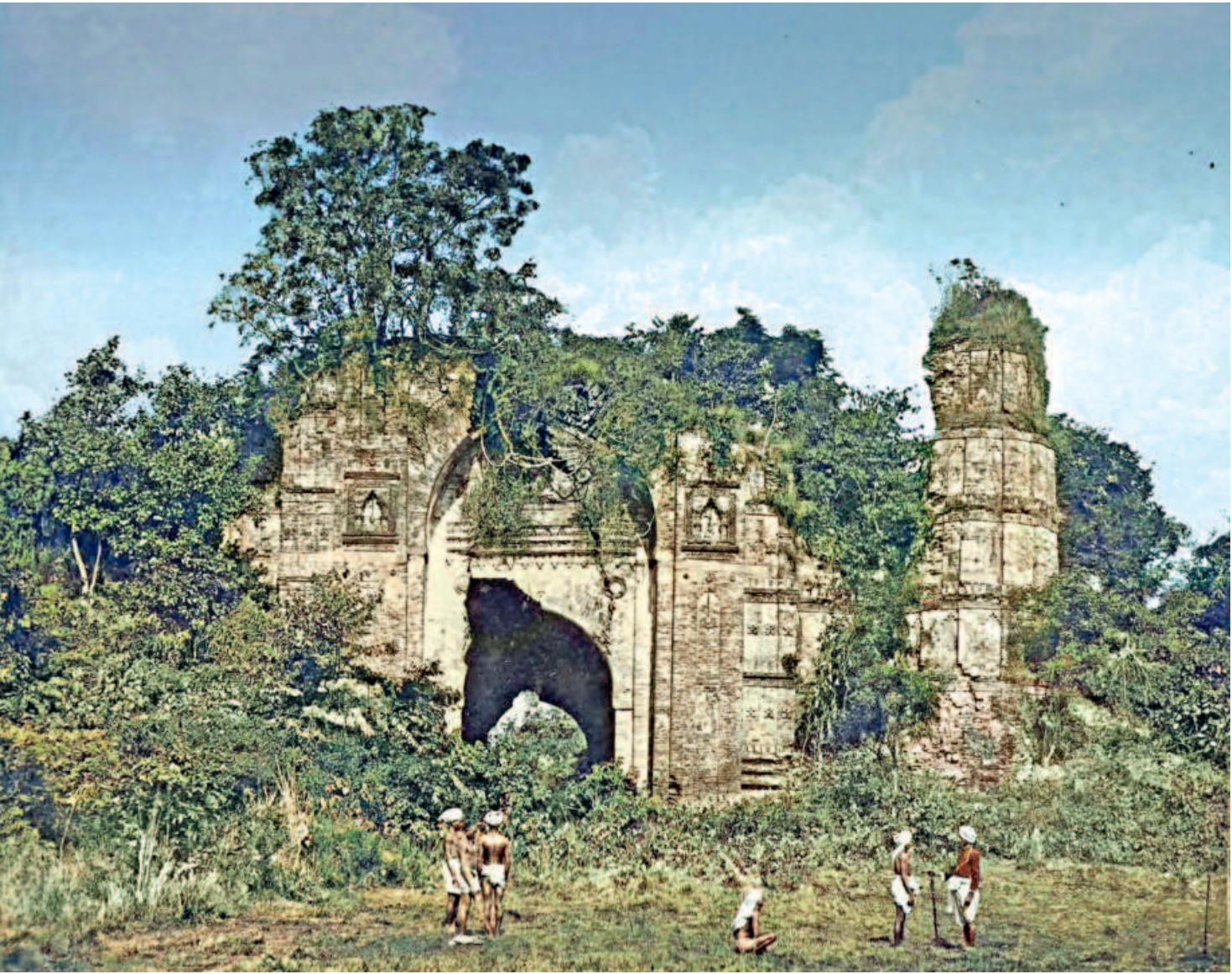
The Dakhil Gate at Gaur, photographed in mid-nineteenth-century colonial India. Once the capital of Bengal, Gaur was severely affected by the earthquake of 1505, which altered the course of the Ganges river system, created malarial swamps and contributed to the city’s eventual abandonment.
