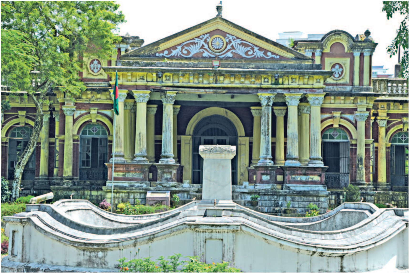
The empty pedestal at Shoshi Lodge in Mymensingh, where a statue of Venus was heavily vandalised and damaged on August 5, 2024.
