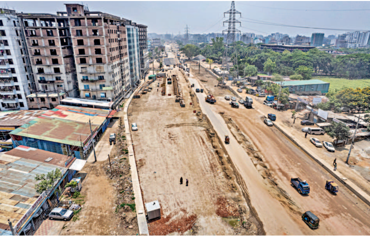
Vehicles ply this under-construction road in the capital's Hazaribagh area as work on the 8-lane Dhaka Inner Circular Ring Road project progresses rapidly. Stretching from Gabtoli to Postogola via Hazaribagh and Kamrangirchar, the mega project is expected to help ease Dhaka's chronic traffic congestion and improve the city's internal transport system once completed. The photo was taken yesterday.
