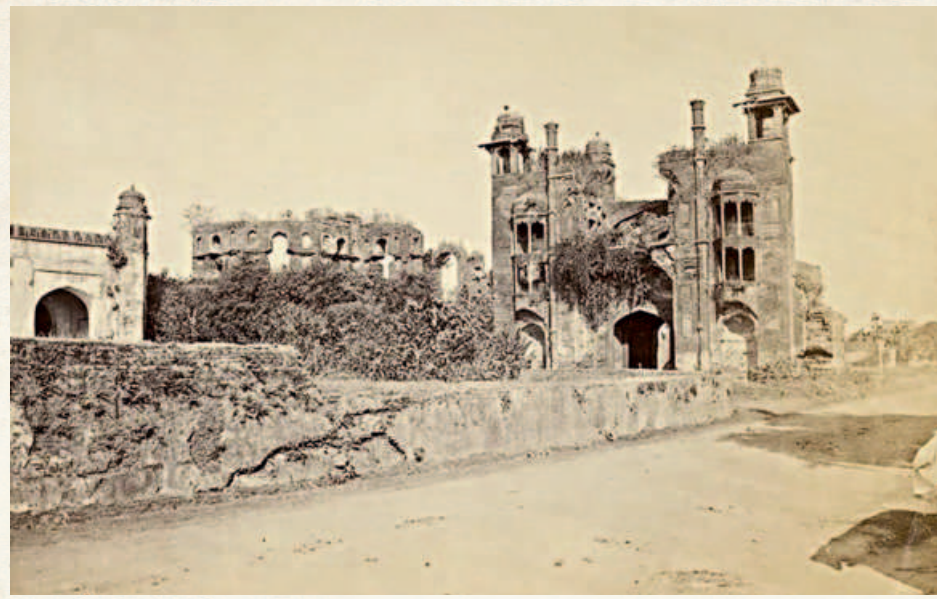
A view of the southern gate of Lalbagh Fort in 1875, nearly two decades after the fierce Battle of Lal Bagh during the Uprising of 1857.
