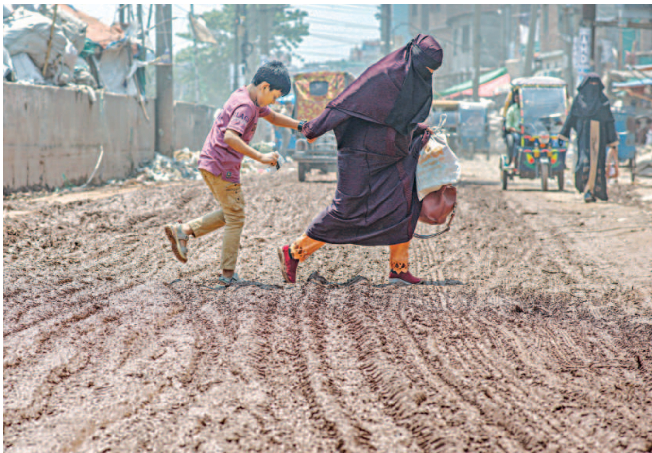
A woman and her son carefully tiptoe through a muddy section of the Sadarghat-Gabtolli Beribadh road in Dhaka's Alir Ghat area. Residents suffer as the dilapidated road becomes nearly impassable during and after rain. The photo was taken recently.
