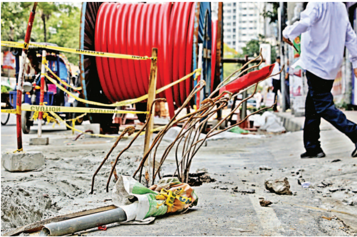
Rods protrude from a temporarily sand-filled section of a road in the capital's Segunbagicha area following underground cable installation work by the Dhaka Power Distribution Company. The absence of proper safety measures poses risks to pedestrians, especially at night. The photo was taken yesterday.
