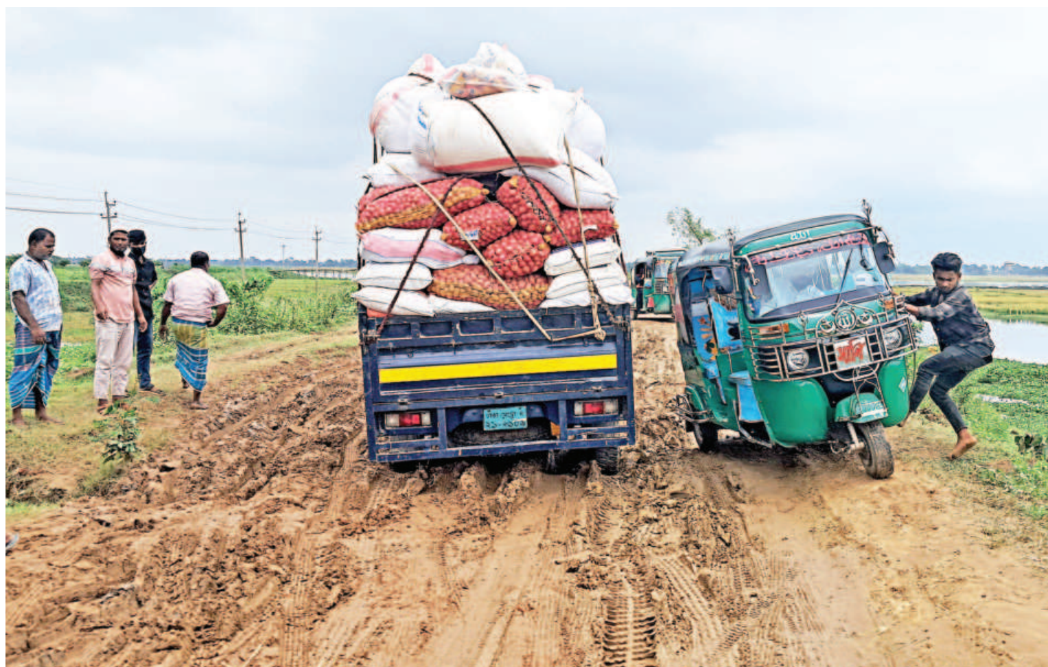
Vehicles struggle through thick mud at the Boalia canal stretch of the Shimna-Brahmanbaria road, where delays in a key bridge project have left approaches nearly impassable. The section regularly traps traffic, causing long jams and severe suffering for commuters between Brahmanbaria town and Bijoy Nagar upazila. The photo was taken recently.
