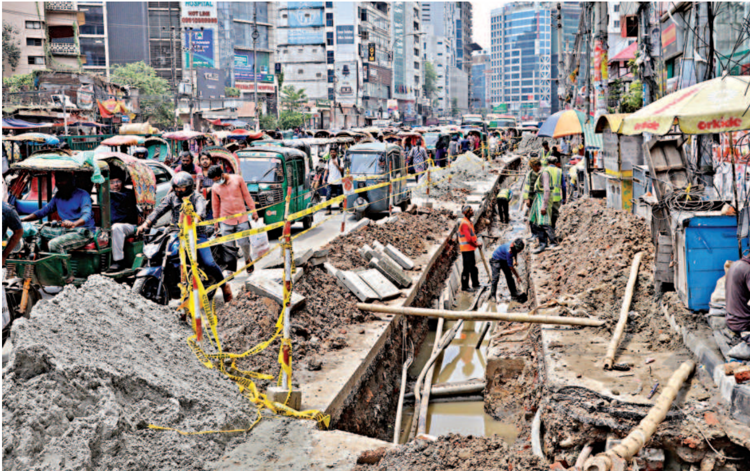
Commuters endure severe traffic congestion as underground cable installation work by the Dhaka Power Distribution Company Limited narrows the main road in the capital's Shantinagar area. The photo was taken yesterday.
