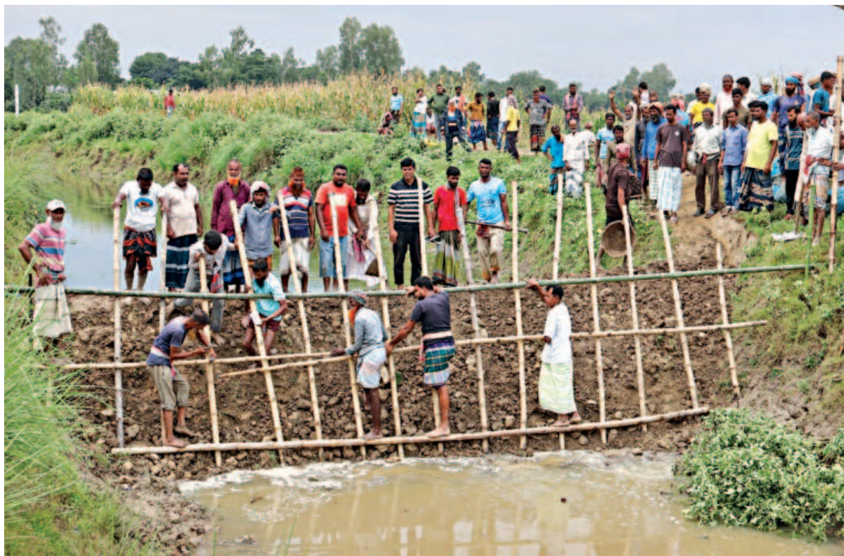
Villagers build a temporary earthen embankment in the Dahapara area of Singra upazila, Natore, to keep floodwaters out of their paddy fields. The photo was taken recently.
