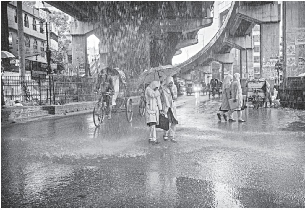
Rainwater cascades from the Muradpur-Lalkhan Bazar flyover in Chattogram during a recent downpour, as faulty drainage causes runoff to spill directly onto the road below, soaking pedestrians and disrupting traffic along the busy stretch.
