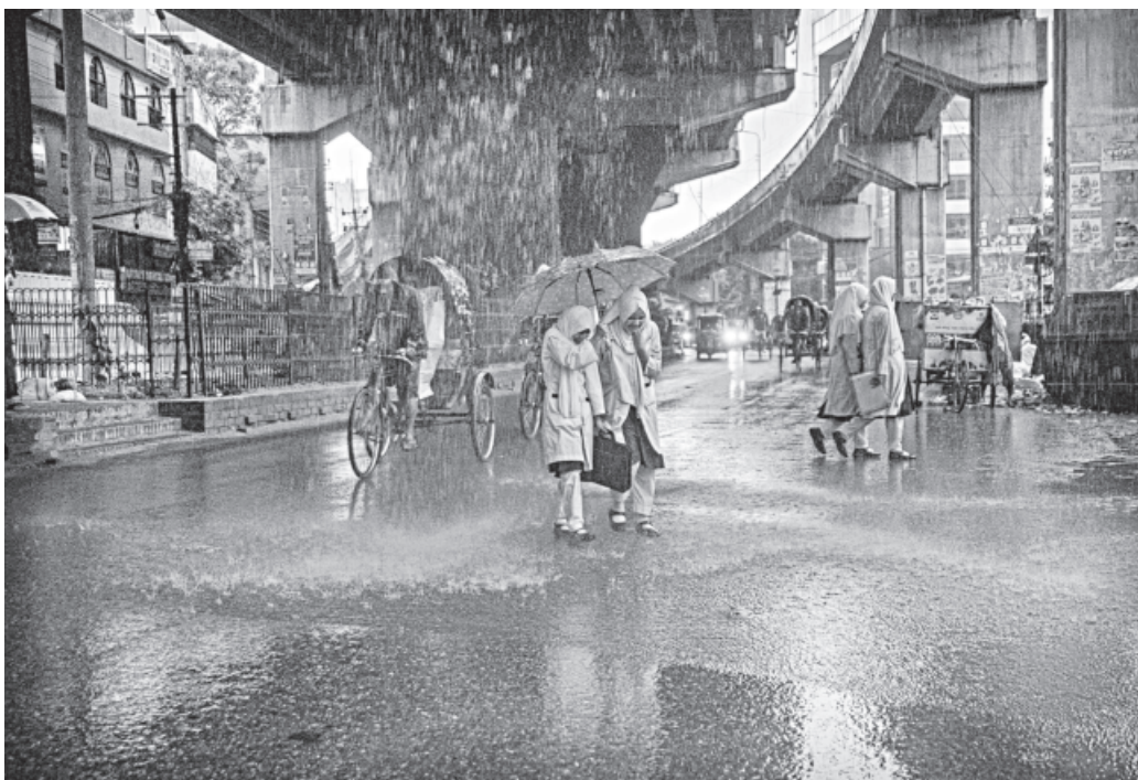
Rainwater cascades from the Muradpur-Lalkhan Bazar flyover in Chattogram during a recent downpour, as faulty drainage causes runoff to spill directly onto the road below, soaking pedestrians and disrupting traffic along the busy stretch.
