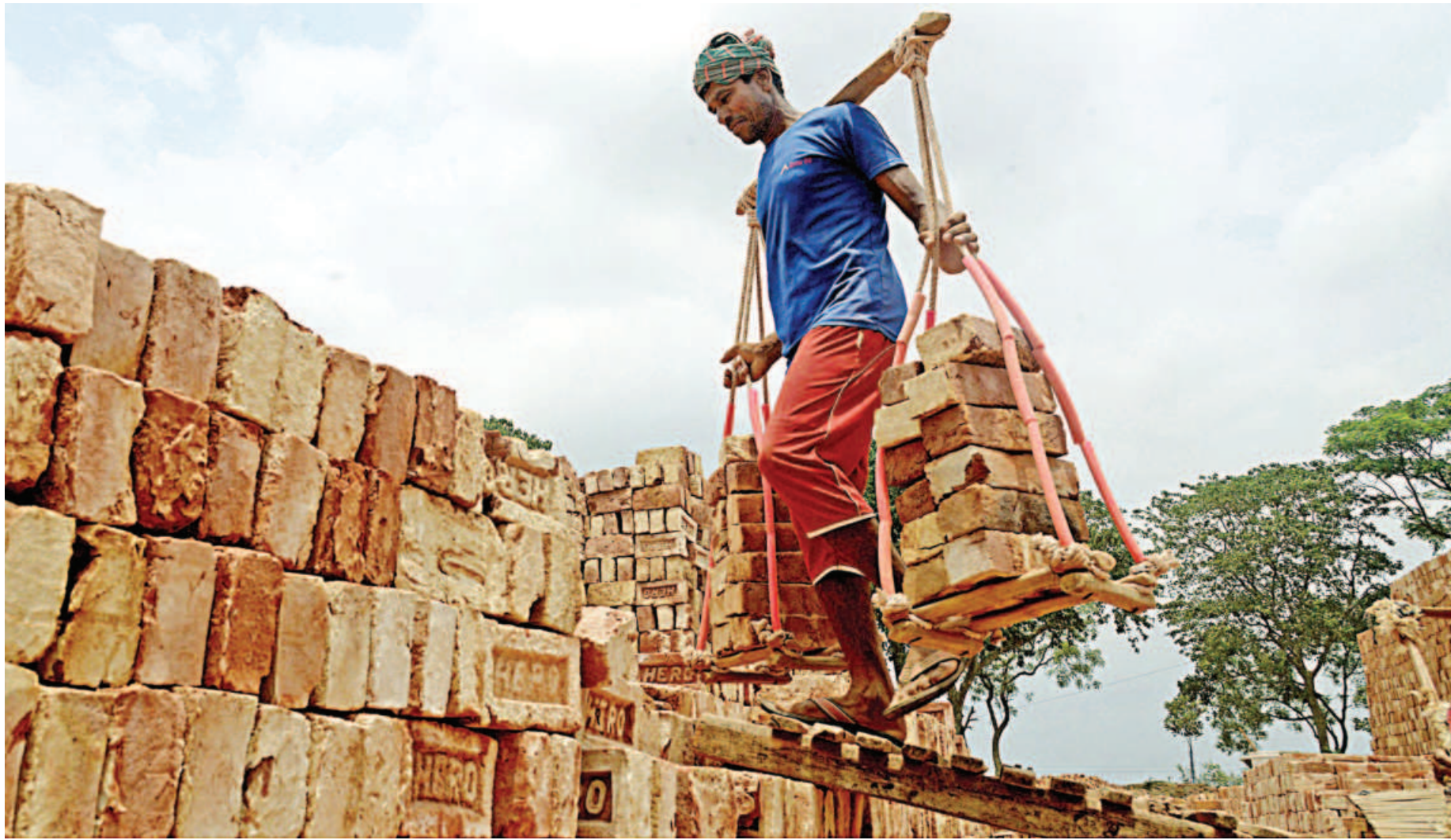
A kiln worker carefully carries bricks across uneven stacks in Manda upazila of Naogaon, doing a risky and physically demanding job for a daily wage of around Tk 600-Tk 700. The photo was taken yesterday, ahead of International Workers' Day being observed today.
