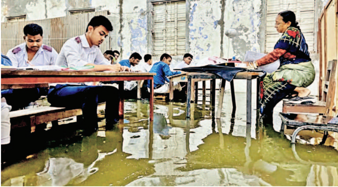
SSC examinees at Comilla Ishwar Pathsala High School centre sit either with their feet raised on benches or just submerged as rainwater floods the exam hall yesterday afternoon. The invigilator is also perched on her chair, while dirty drainwater floats through the rooms after an hour and a half of heavy rain left much of Cumilla city waterlogged. PHOTO: COLLECTED
