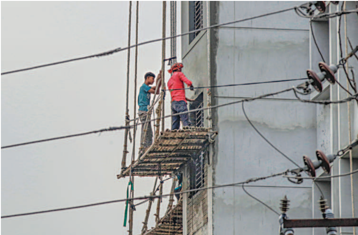
On a suspended bamboo scaffold six floors above the ground, two construction workers plaster the side of a high-rise government building. Without any safety harnesses or protective gear, the risk of a fall is serious. The photo was taken yesterday near the capital’s Tejgaon Truck Stand area.
