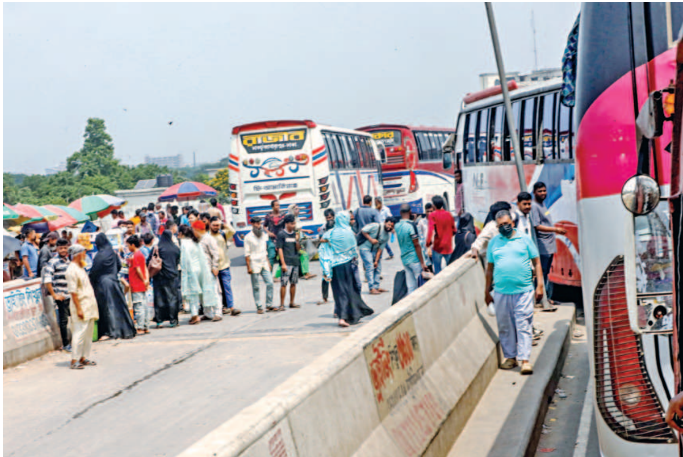
Bus operators have illegally set up counters on the Uttara-Abdullahpur flyover in the capital. This is effectively choking the high-speed corridor, as buses stop in the middle of the road to let passengers get on and off. The flyover was built to spare passengers from such congestion. The photo was taken yesterday.
