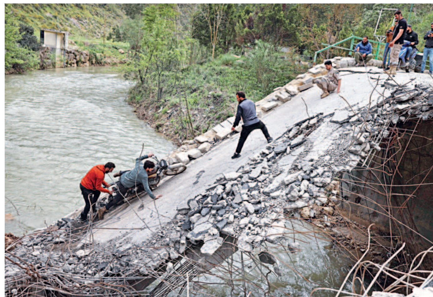
People help a motorcyclist cross a bridge damaged in an earlier Israeli strike, during a 10-day ceasefire, in Zraieh, southern Lebanon, yesterday.
