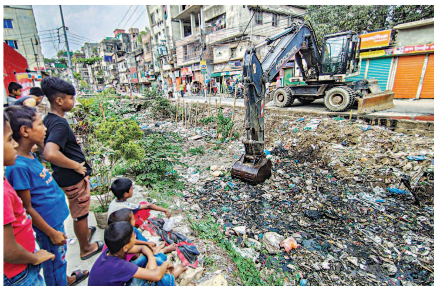
An excavator removes heaps of solid waste from the Kazla canal in the Jatrabari area of Dhaka yesterday afternoon. While the Dhaka South City Corporation has undertaken the project to improve drainage and reduce waterlogging, numerous illegal structures remain along the banks of the canal, complicating the restoration efforts.
