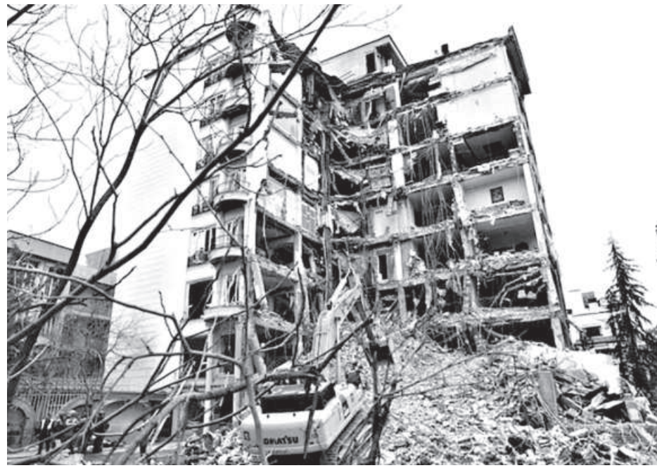
A view of a residential building damaged by a strike, amid the US-Israeli conflict with Iran, in Tehran, Iran, March 23, 2026.
