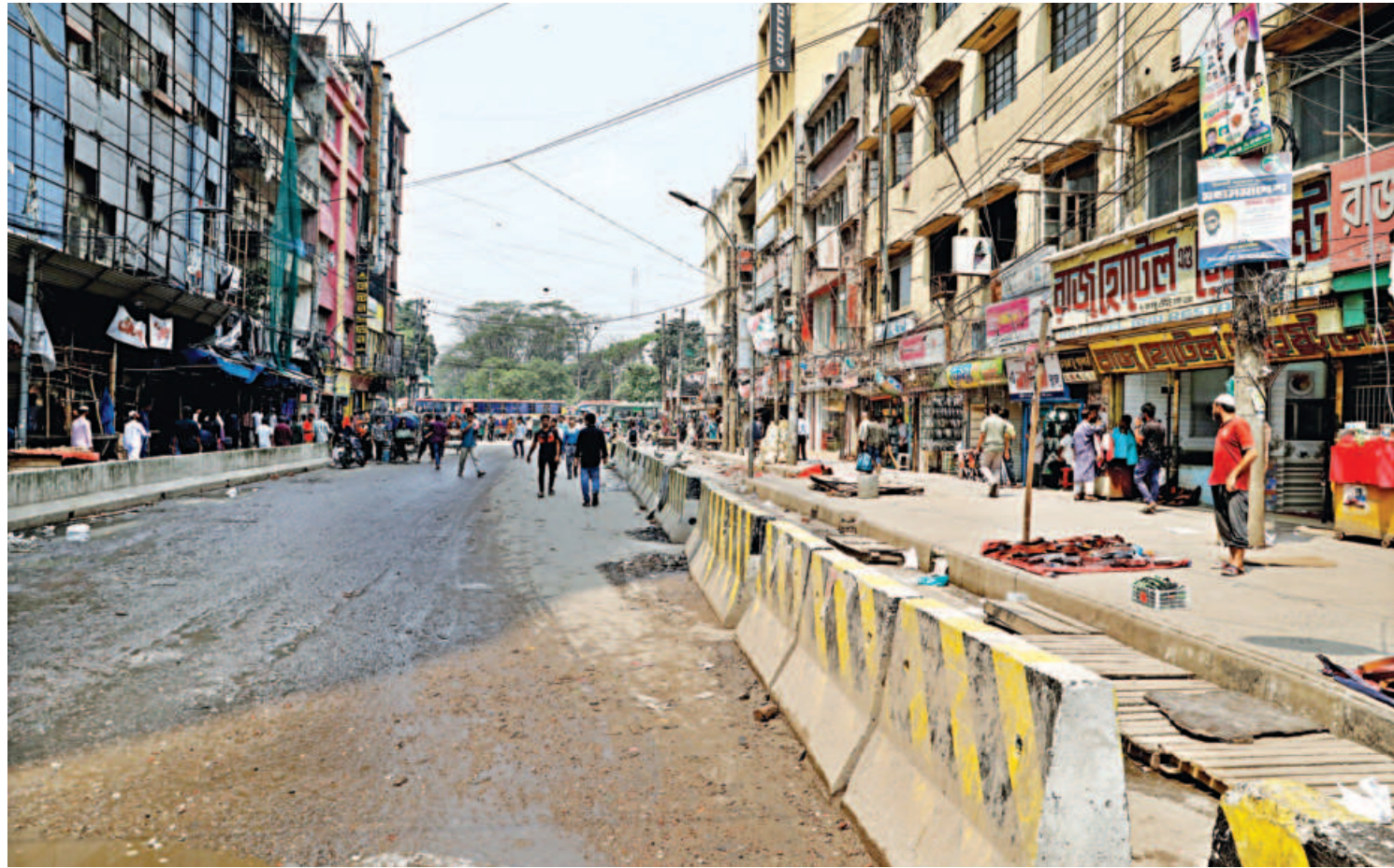
Once crowded with makeshift hawkers' stalls, Shaheed Abrar Fahad Avenue -- formerly Bangabandhu Avenue -- in the capital's Gulistan now appears relatively empty. Law enforcers had warned of an ongoing eviction drive by the DSCC to reclaim encroached footpaths and roads, prompting hawkers to voluntarily close their shops and leave the area. The photo was taken yesterday.
