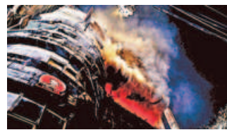
The investigation also found that stairways and emergency exits were obstructed by gas cylinders and other materials, significantly increasing the death toll.
