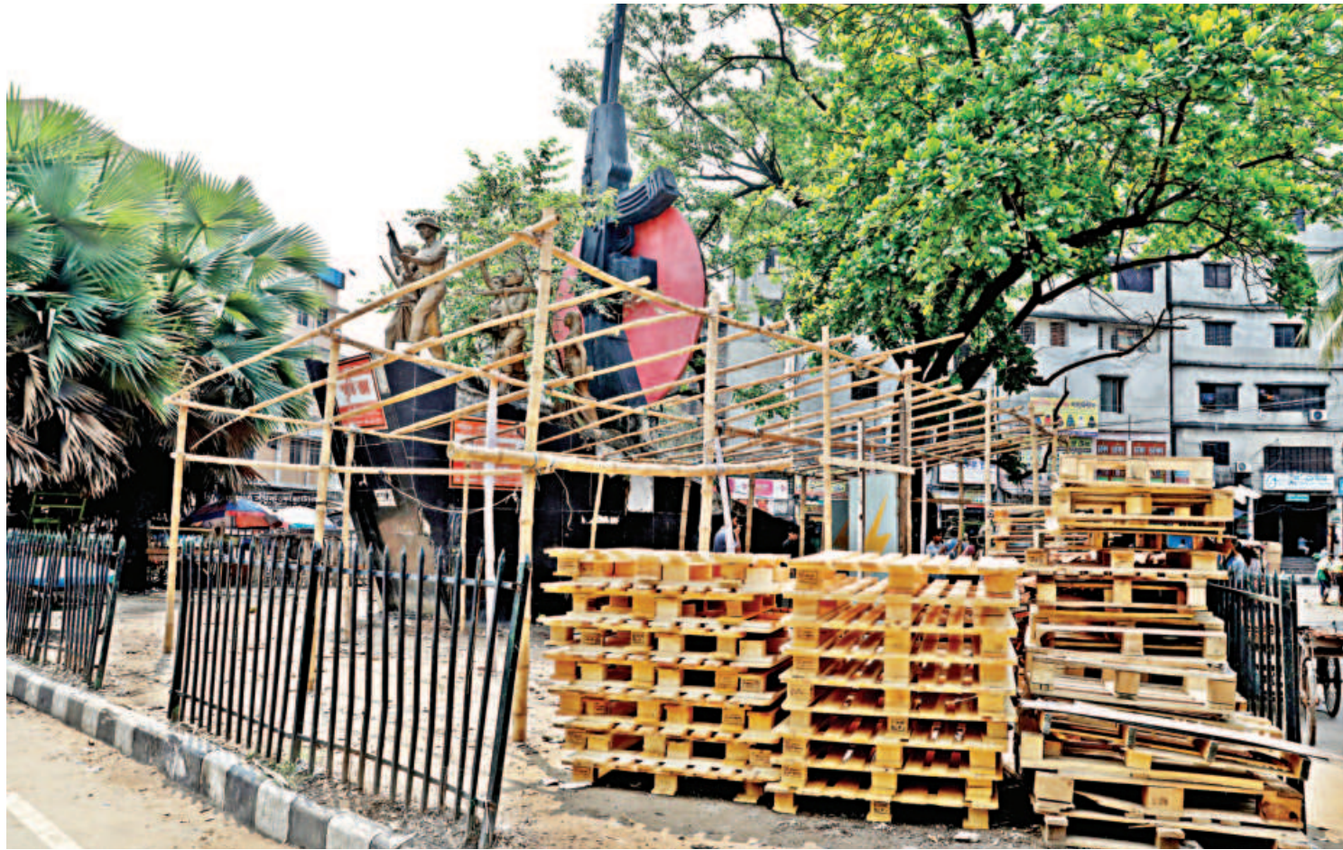
Wooden structures and a makeshift bamboo shack turn the Shaheed Selim-Delwar Memorial into an eyesore, showing clear neglect and disrespect. The site near Dhaka University's Amar Kushey Hall is now encroached upon by roadside businesses. HM Ibrahim Selim and Kazi Delwar Hossain were killed when a police truck rammed into a student protest against HM Ershad's autocratic regime in Gulistan in 1984. The photo was taken yesterday.
