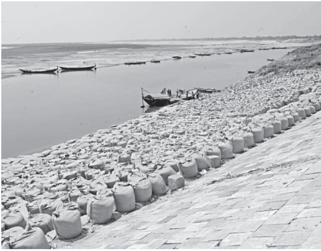
Sandbars have emerged across much of the western bank of the Padma River in the Aibadh area of Rajshahi city, making it appear fragmented into narrow canals. Boat movement has come to a halt, while the Water Development Board has begun work beneath the city protection embankment ahead of the monsoon. The photo was taken recently.
