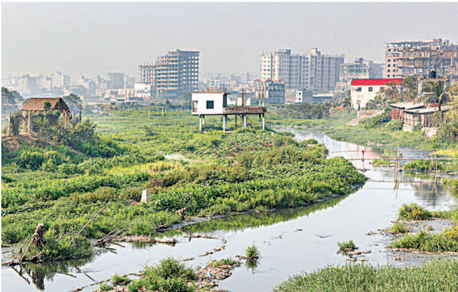
Illegal structures built haphazardly on Satarkul canal have narrowed the once wide waterbody, linked to the Balu river, in the city's Badda. This photo was taken recently.
