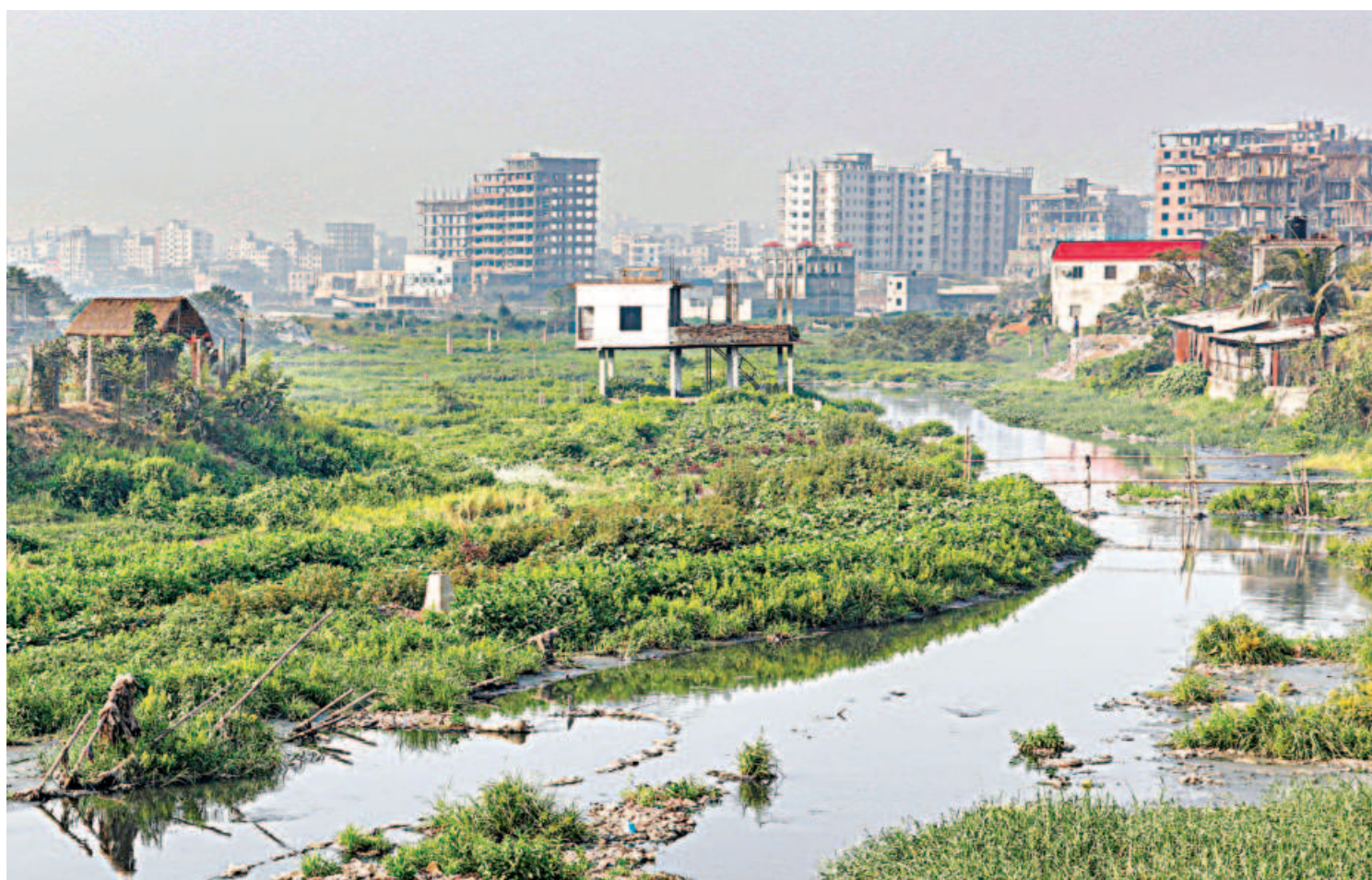
Illegal structures built haphazardly on Satarkul canal have narrowed the once wide waterbody, linked to the Balu river, in the city's Badda. This photo was taken recently.
