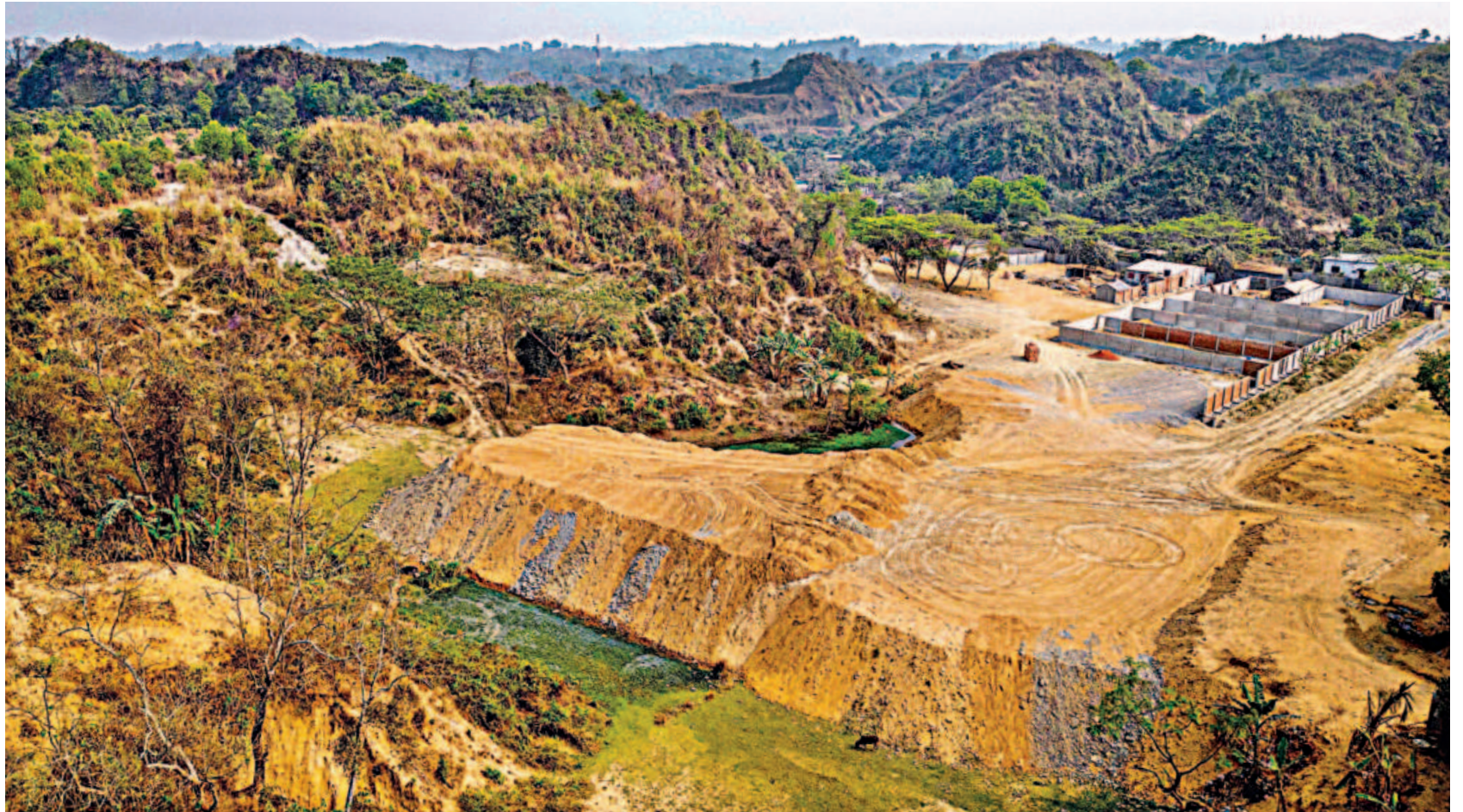
Markets, roads, and homes are being built by cutting the hills of Jungle Salimpur at Alinagar in Sitakunda, Chattogram. The razed hills of the area lay bare the environmental impact of encroachment. This photo was taken recently. PHOTO: RAJIB RAIHAN
