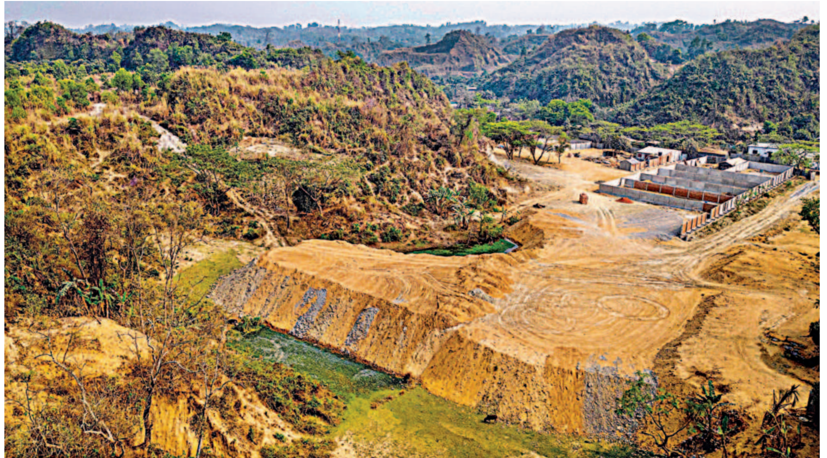
Markets, roads, and homes are being built by cutting the hills of Jungle Salimpur at Alinagar in Sitakunda, Chattogram. The razed hills of the area lay bare the environmental impact of encroachment. This photo was taken recently.
