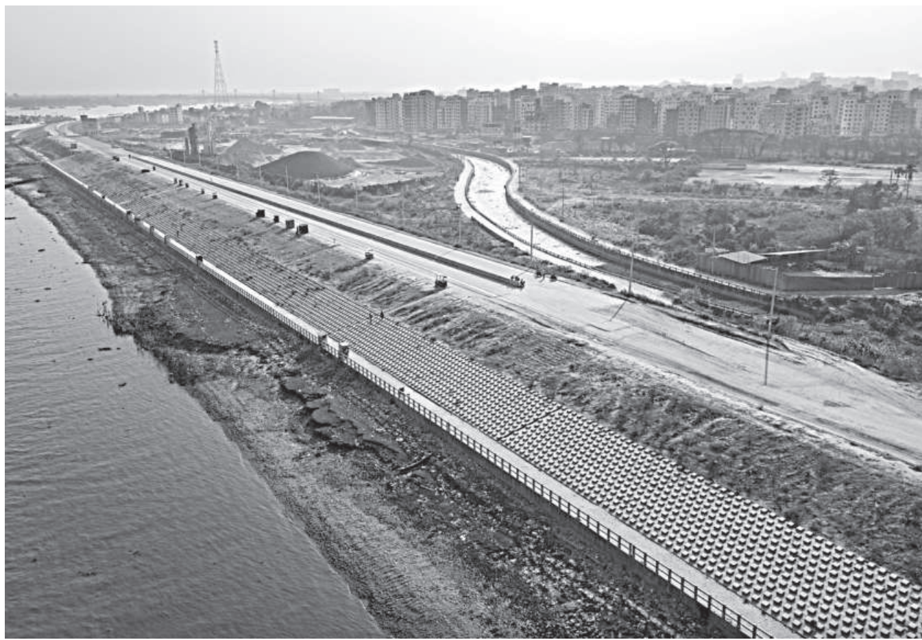
Work on the Kalurghat-Chaktai road and dyke project in Chattogram is still underway, nearly nine years after it was launched in July 2017 with a completion target of three years.
