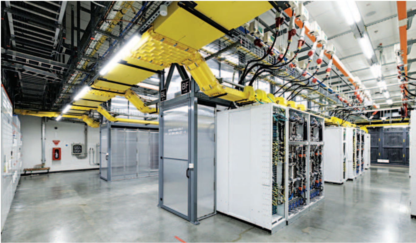
In this photo, racks of graphics processing units with a closed-loop liquid cooling system are seen inside an operational Microsoft data centre in Karawang, West Java.
