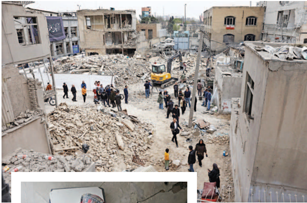
Residents walk past the rubble of buildings hit by an airstrike in Tehran yesterday. Inset, a woman picks up belongings inside a house that was damaged by a strike in Tehran. Iran yesterday warned countries against getting involved in its war with the United States and Israel, after President Donald Trump urged world powers to escort oil tankers through the Strait of Hormuz choke-point in the Gulf.
