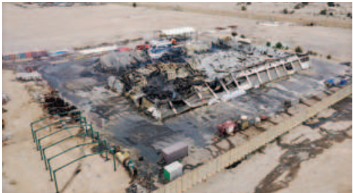
PHOTO: REUTERS A damaged compound housing offices and warehouses used by a US firm, in Iraq.
