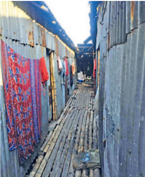
A narrow lane in a Shyampur informal settlement: tin walls press close on both sides, laundry strung overhead, and no through ventilation.
