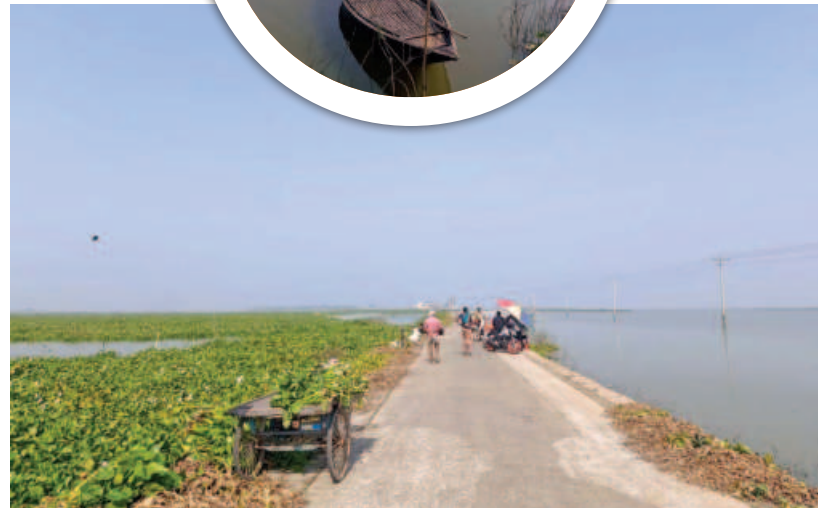
Several roads have split the waterbody over the last decade.
