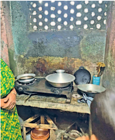
A cooking space in a Dakshinkhan informal settlement: a gas burner on a soot-darkened ledge, walls blackened with years of combustion residue, and a lattice vent as the only source of air.
