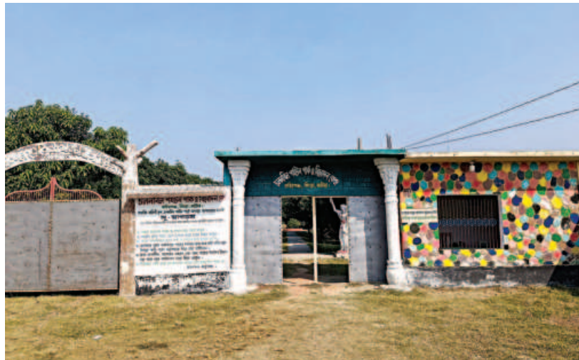
Structures like these have further exacerbated the wetland's demise.
