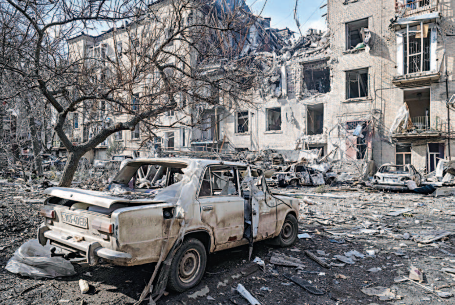
Burned-out cars lie beside a damaged residential building after a Russian air strike in Druzhkivka, Donetsk region, Ukraine on Monday, in this handout from Ukraine’s 93rd Kholodnyi Yar Brigade.
