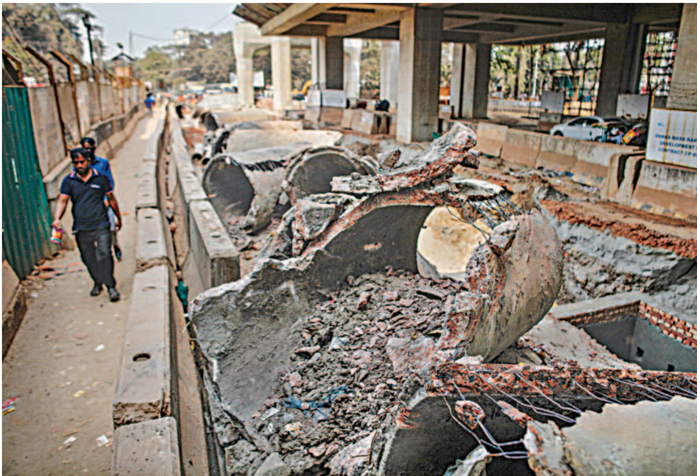
This stretch of the road opposite Kamalapur Railway Station in Dhaka has remained dug up for over a month, causing inconvenience to commuters and pedestrians. Dhaka Mass Transit Company Ltd is repairing drainage lines damaged during its construction, but work has progressed slowly. The photo was taken recently.
