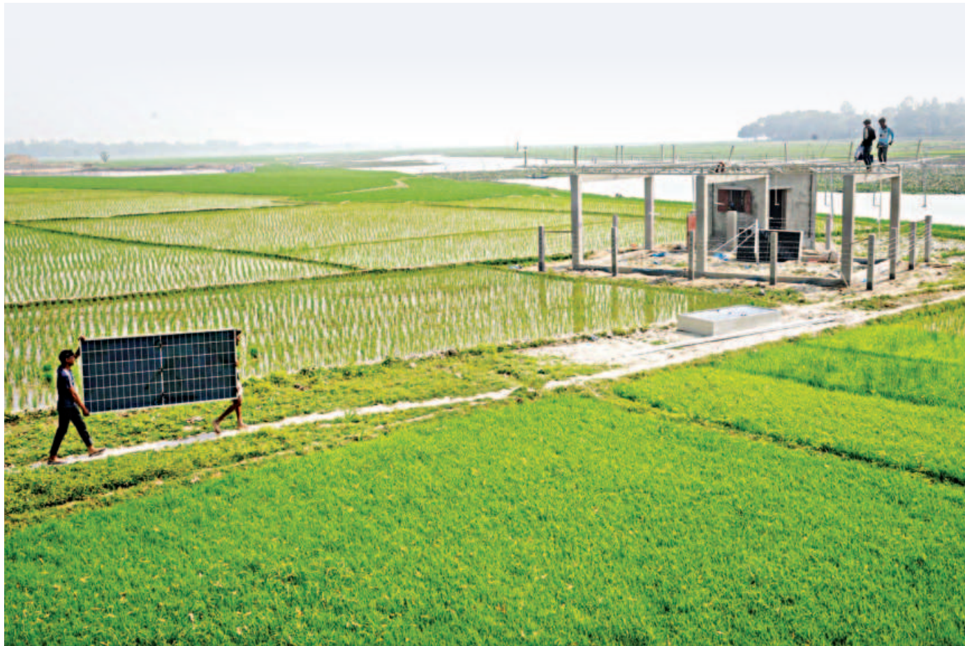
Solar-powered irrigation systems are being installed across different upazilas of Naogaon. Farmers are now using such renewable energy sources to draw water from underground sources to meet irrigation needs. The photo was taken yesterday in the Delwarbari area of Manda upazila, Naogaon.
