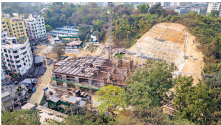
The work for 'China-Aid Project of Burn Unit of CMCH' continues in the city's Goachi Bagan area.
