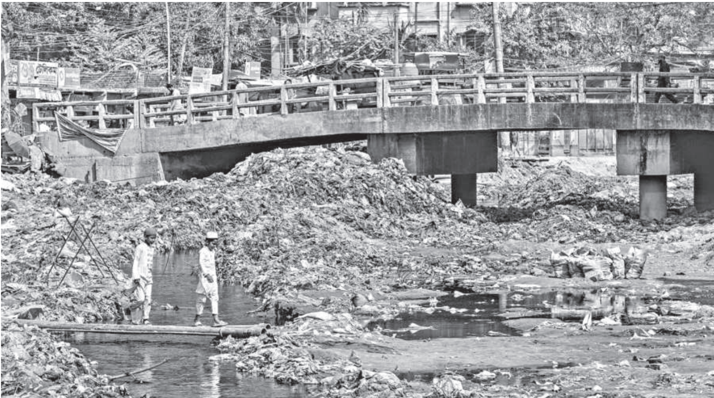
The Subhadya Canal in Keraniganj, Dhaka is one of many across Bangladesh that are on the verge of dying and are in desperate need of excavation to restore water flow.
