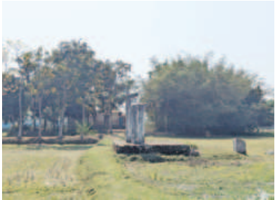
The dilapidated shaheed minar built in memory of Abdul Jabbar in Shimulkuchi village in Mymensingh's Haluaghat upazila. There is no road leading to the shaheed minar and his family home.
