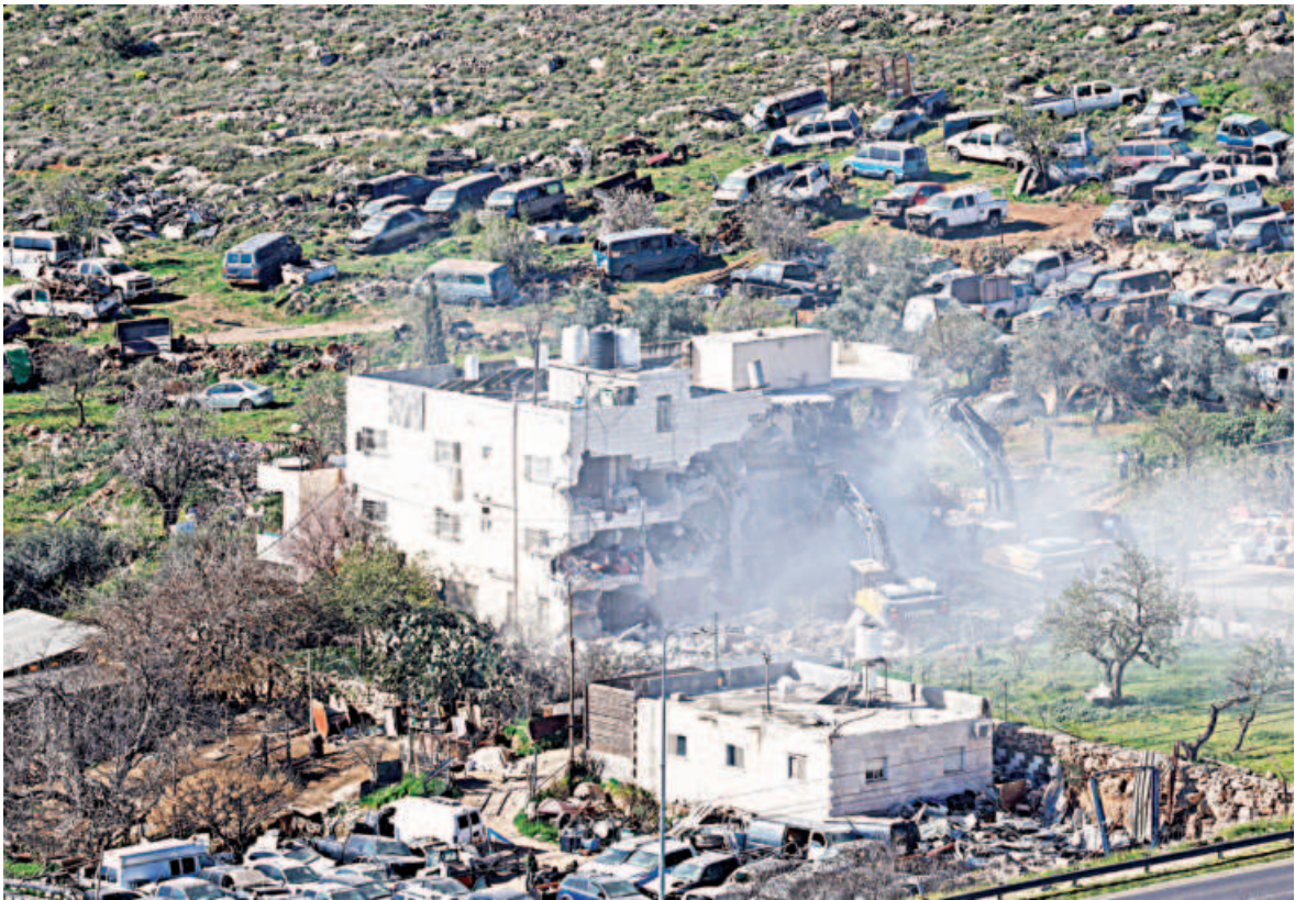
Heavy machinery demolishes a Palestinian building near Hebron in the Israeli-occupied West Bank yesterday. A senior Israeli far-right minister vowed to encourage “emigration” from the Palestinian territories, despite mounting criticism of recent measures tightening Israel’s control over West Bank. PHOTO: REUTERS
