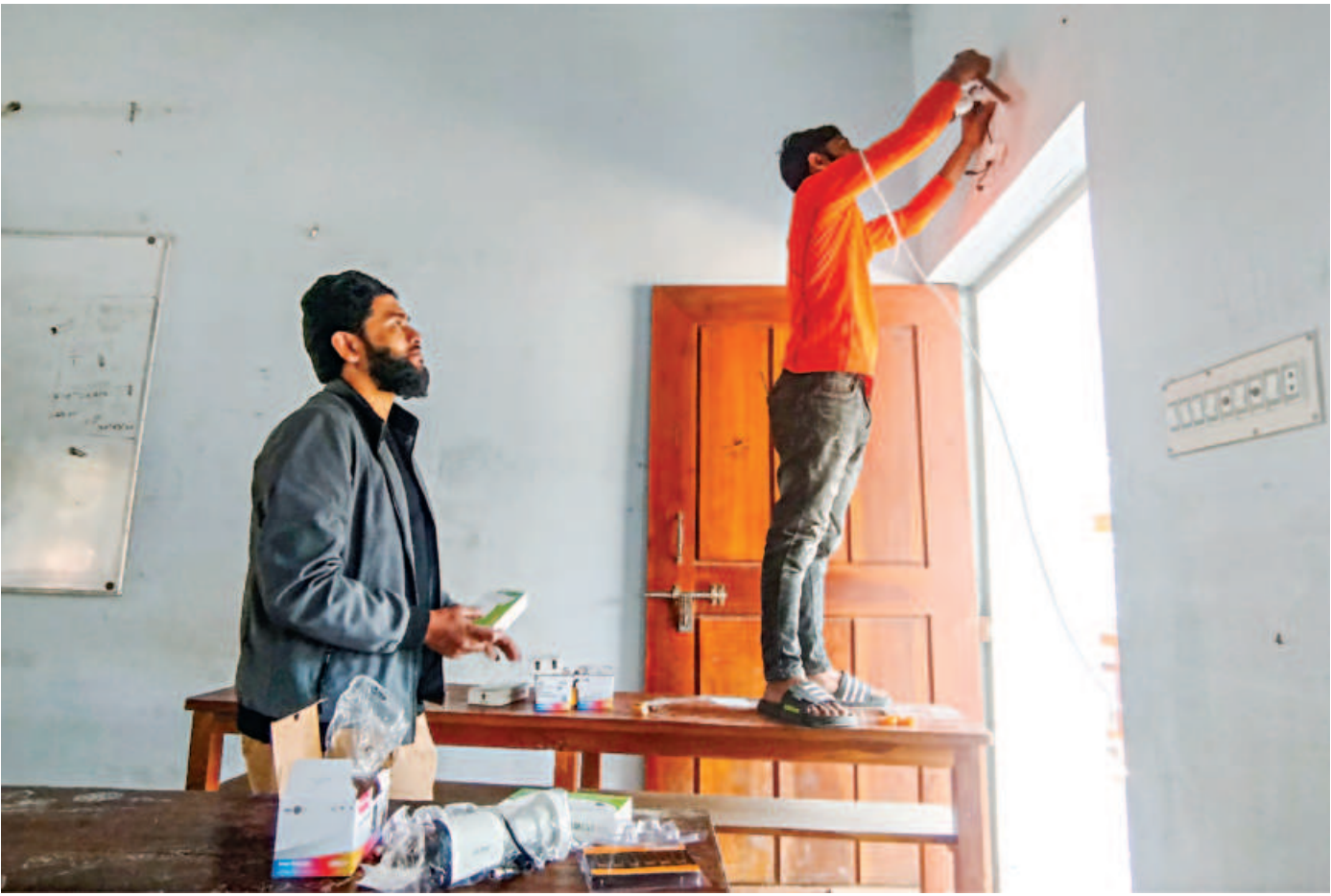
Workers set up CCTV cameras at Iqbal Nagar Secondary School voting centre in Khulna city yesterday ahead of the national polls. The Election Commission took the initiative to install cameras at the polling stations to monitor voting.
