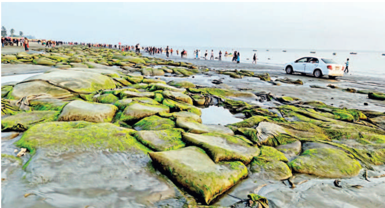
Around five- to six-year-old sand-filled geo-bags lie along Kuakata Sea Beach, with algae growing on them over time. Although installed to prevent beach erosion, the geo-bags have become hazardous as algae and dents make them slippery and unsafe for locals and tourists. The photo was taken recently.
