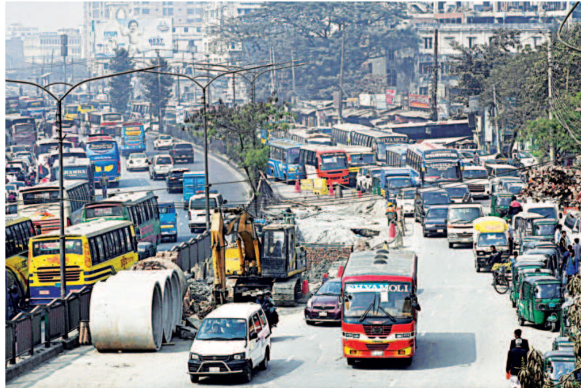
Dhaka North City Corporation is digging up part of the lane leading from Gabtoli to Technical to install sewage pipes. The work, which occupies half of this busy entry point to the capital, leaves vehicles stuck for long periods. The photo was taken yesterday.
