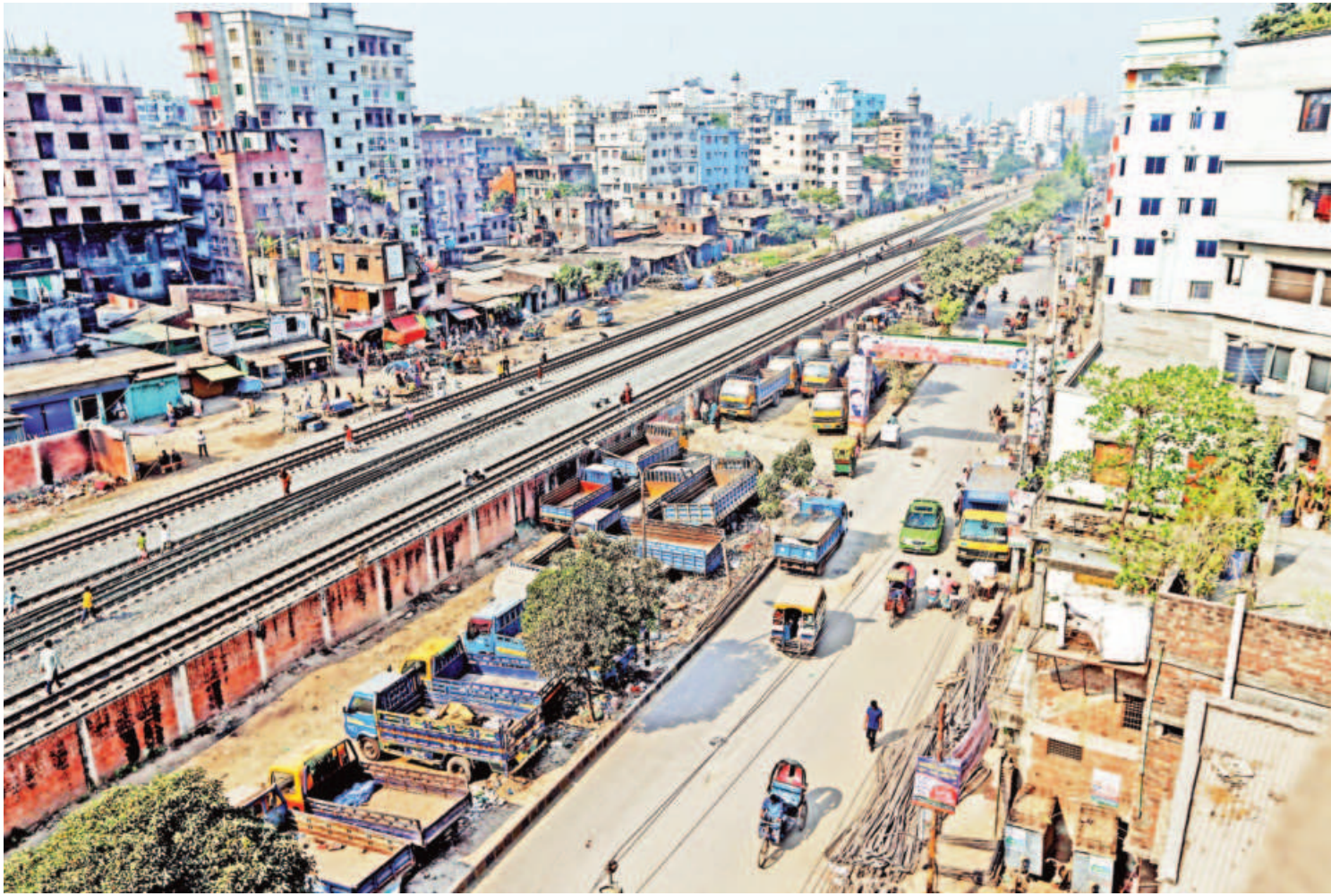
The Dayaganj-Jurain Road has been in a neglected state for a long time after Bangladesh Railway built a boundary wall along the rail line, significantly narrowing the road. Due to reduced width and severe deterioration, the road has become a struggle for commuters.
