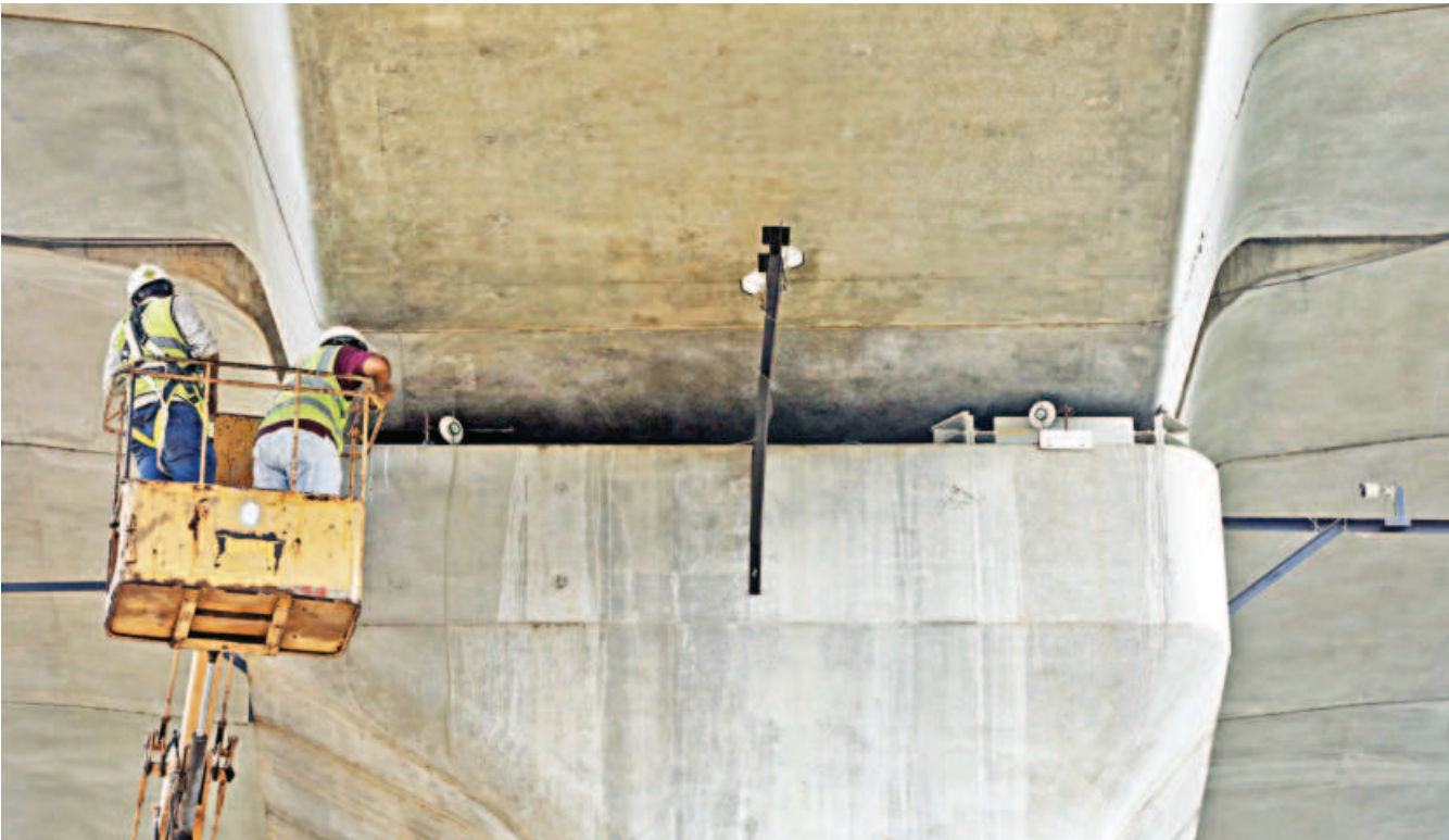
Surveillance cameras are being installed on a metro rail pillar to monitor the condition of bearing pads near the Farmgate Metro Rail Station. The photo was taken yesterday.
